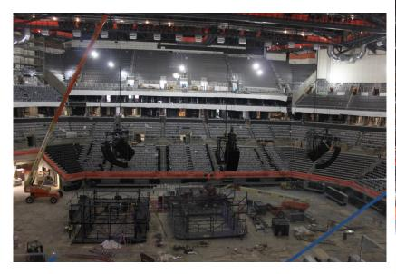
Polar Focus collaborated with Dave Potts of Parsons Electric on this project. There were six line array clusters with 10 EAW KF740 and 4 EAW SBS1001, each totaling 2385 lbs per cluster.
