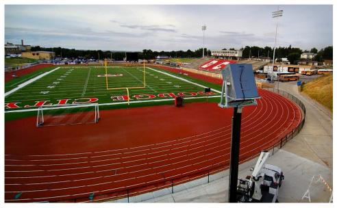
McClelland Sound contacted us for a custom bracket with full tilt control for the amazing 720 pound Danley Sound Labs, Inc. JH-90 speaker. The Danley JH-90 "Jericho Horn" has six 18" drivers, six 6" midrange drivers and three coaxial high frequency drivers with 1.4" exits coupled to Danley's patented layered high frequency combiner.
