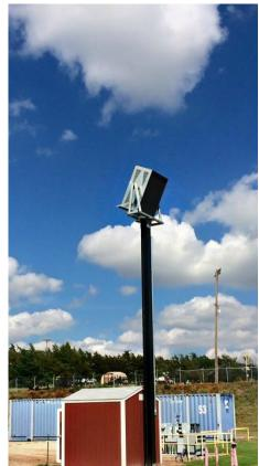
Once mounted to the top of this W10x49 column, the speaker has full pan and tilt control and can be locked into position.
