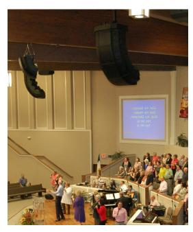
Additional speakers from Bose were used as choir fills. Mark chose Polar Focus for our family of wood beam brackets for super clean installation. Polar Focus also supplied an aftermarket line array frame for the Bose RoomMatch with integral tilt control and a full range of accessories. Using a Custom Beam Attachment to connect to the wood beams with a structural extension post that was also a cable raceway resulted in a very clean and safe installation.
